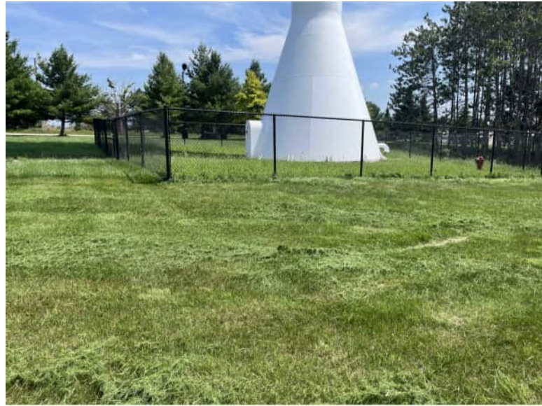
TANK BASE FACING EAST
