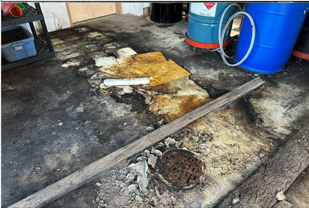
Photo 12: A view of the used frying oil that has spilled onto the floor and entered the floor drain. The entire floor of the shed needs to be degreased/cleaned.
