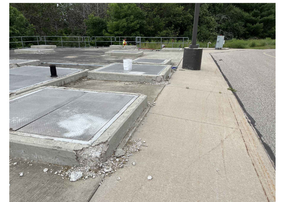
DIGESTER NE CORNER FACING NW
