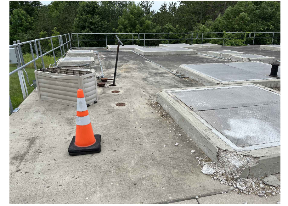
DIGESTER NE CORNER FACING SW
